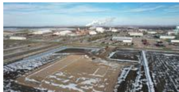
The second building phase of the Ag Innovation Campus is set to begin in spring 2022.
